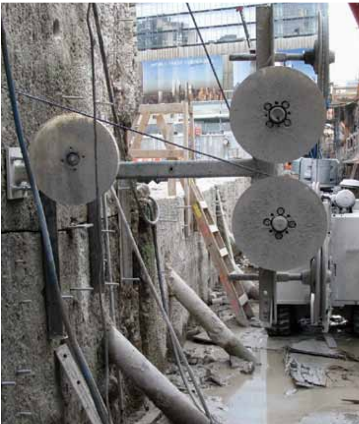
Diamond wire sawing was used to perform the cuts.
