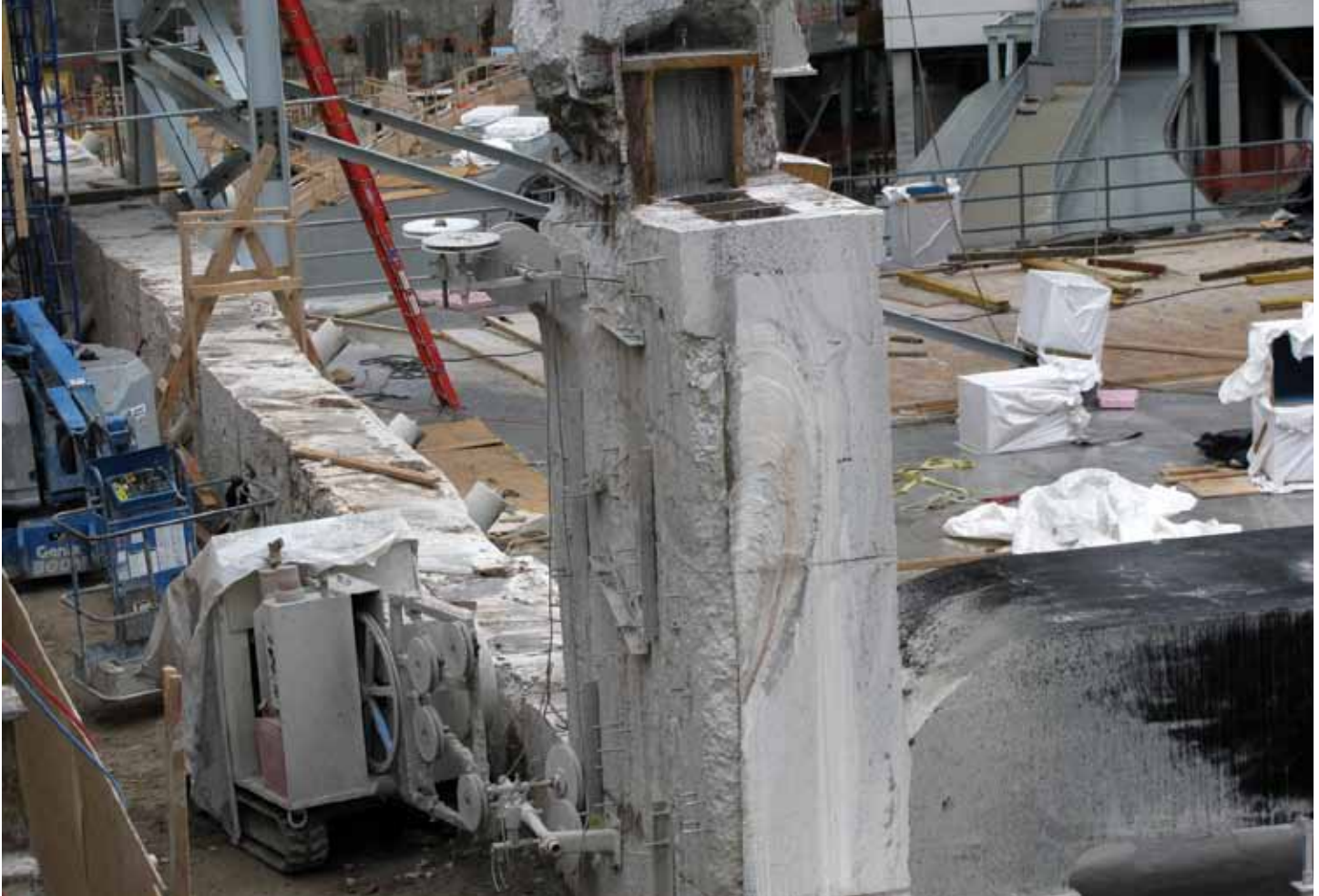
3,200 picking holes were drilled for removal by crane.
