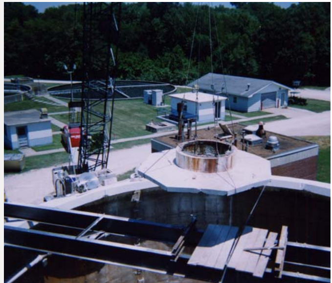
Clockwise from top left: Only one section remains to be cut during phase one of the project. The sections were rigged for removal before the last two cuts were made. The I-Beams that supported the center section can be seen as the final piece of the tank cap is removed. Fall protection was critical throughout the entire job.
