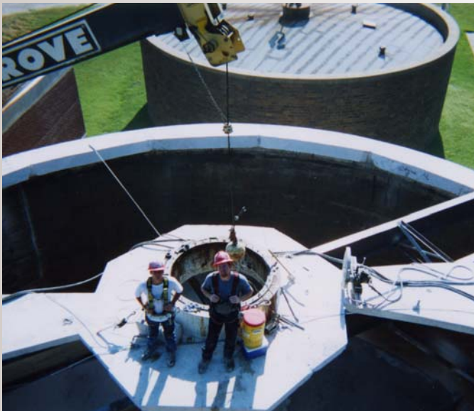
Clockwise from top left: Only one section remains to be cut during phase one of the project. The sections were rigged for removal before the last two cuts were made. The I-Beams that supported the center section can be seen as the final piece of the tank cap is removed. Fall protection was critical throughout the entire job.
