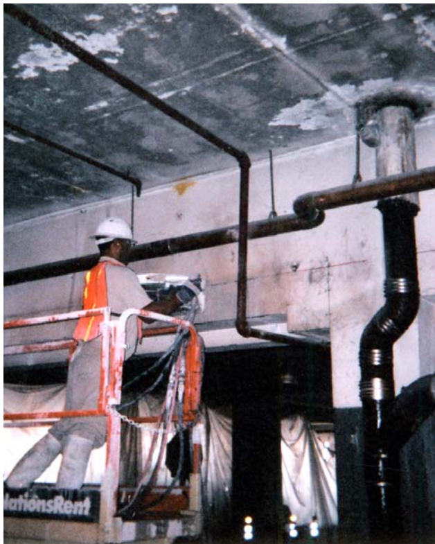
Above: Concrete cutting was needed to remove 15 reinforced concrete beams in one of the airport's infills.
