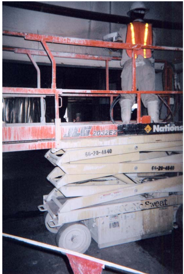
Above: Concrete cutting was needed to remove 15 reinforced concrete beams in one of the airport's infills.
